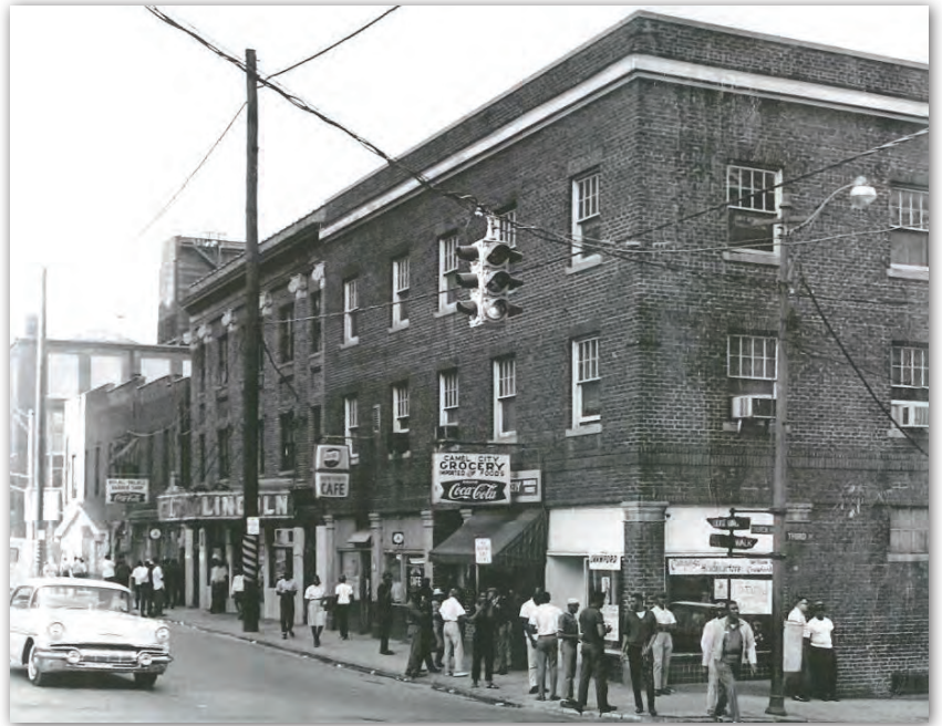
Church and Third Streets, 1966. Photo by Frank Jones. Forsyth County Public Library Photograph Collection, Winston-Salem, NC.
